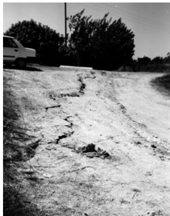
Figure 3: Part of a seismic rupture caused by sinistral strike slip movement.
