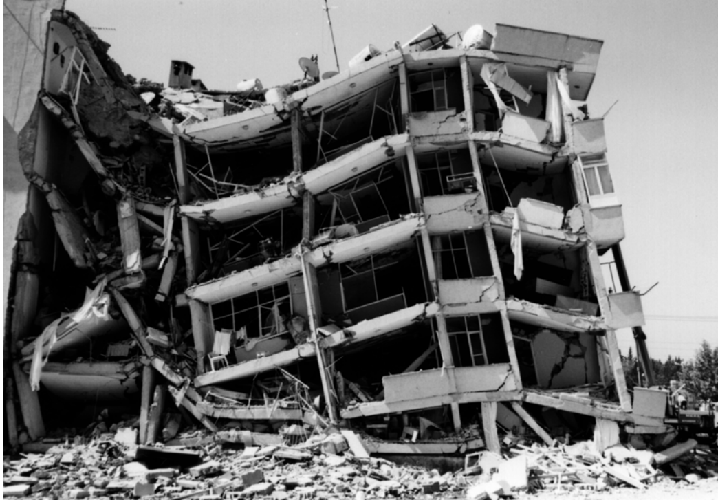
Figure 4: Total collapse of multi-story building at the city of Ceyhan.
