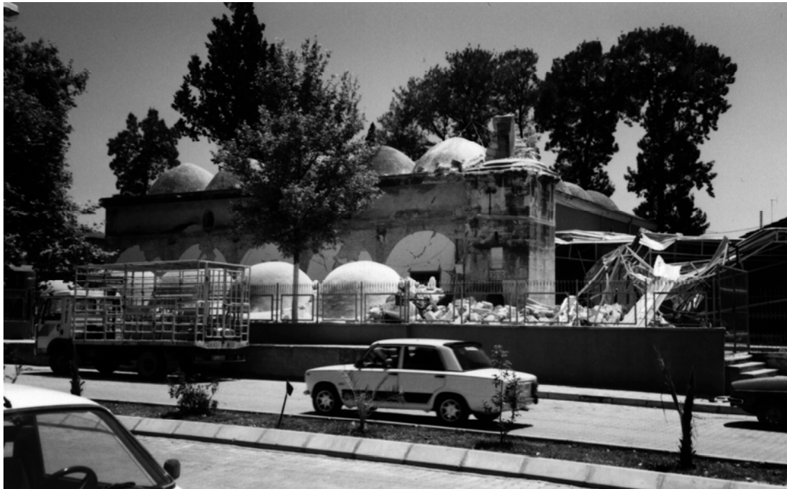
Figure 5: Partially collapsed mosque in the city of Ceyhan.
